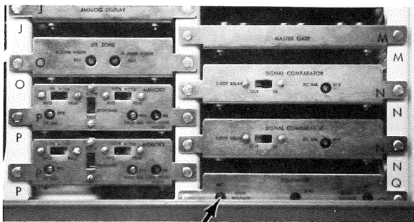
R87 Stop Voltage Cal
