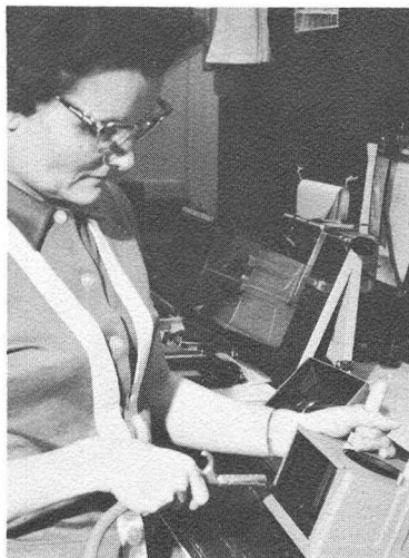
DOROTHY FORNSHELL (Precision Mechanical Assembly) uses air nozzle adaptor to blow lint from C-12 camera case.
