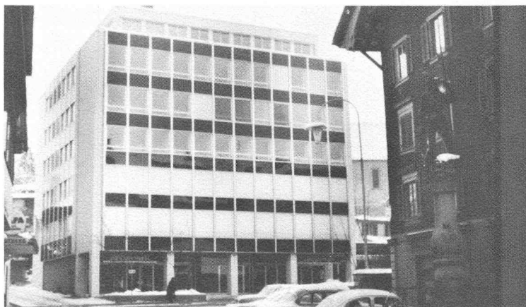
NEW ZUG HEADQUARTERS — Third floor (European style), Zeug-Haus Gasse #9, Zug, Switzerland.
