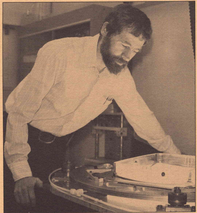
Jerry monitoring the phosphor deposition process on a 19-inch panel.
