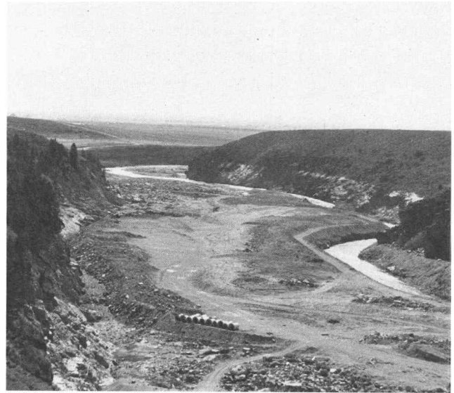
Fig. 15. Faintly visible here, Sugar City lies 11 miles below the dam. On its rush downstream, the surge of water tore out trees and cut away the bank. Below, it spread out into the valley eight miles across, but was still 10 feet high as it inundated Rexburg 15 miles below.
