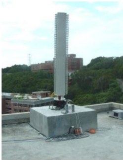
Receiving part of the landfill
