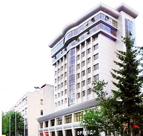
Photo of the building, the construction of which began at LNIRTI.
